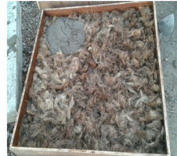
Figure.11 Mortar Placing Above The Palm Fibre
