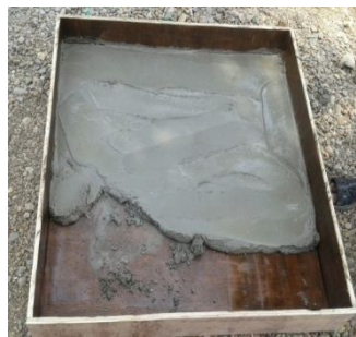
Figure. 10 First Layer Of Mortar
