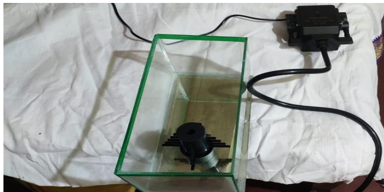
Fig. 3 Final diffused aeration system
