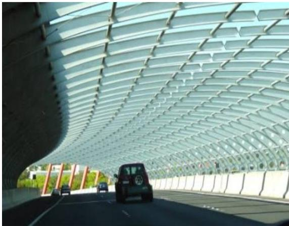
Figure 2: Sound-proofing shed & architecture (Source: Web)
