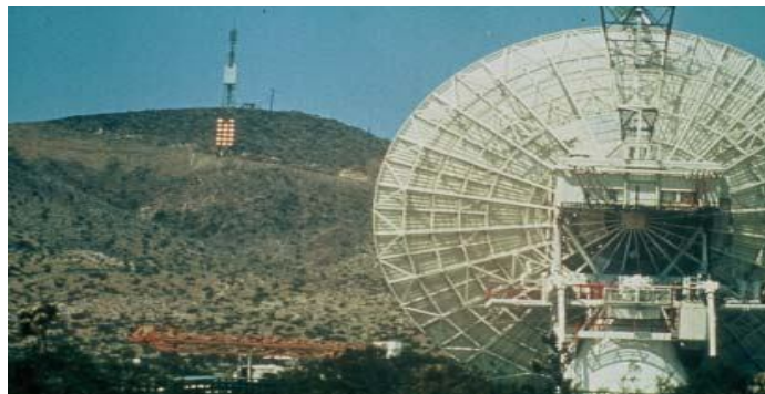
Fig. 7 FIRST GROUND TO GROUND MPT EXPERIMENT AT VENUS SITE OF JPL GOLDSTONE FACILITY
