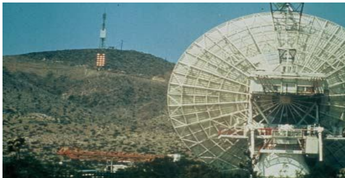
Fig. 7 FIRST GROUND TO GROUND MPT EXPERIMENT AT VENUS SITE OF JPL GOLDSTONE FACILITY
