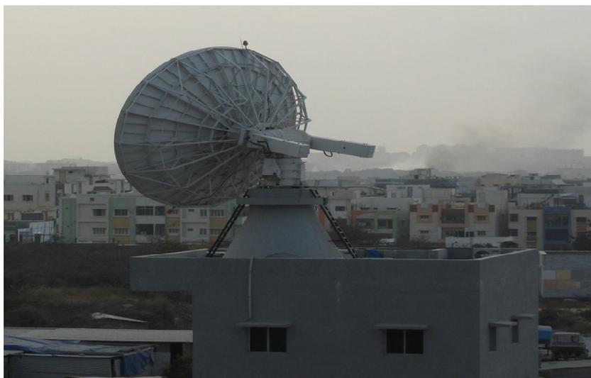
**Figure 1:** X-Band Polar Satellite Antenna
