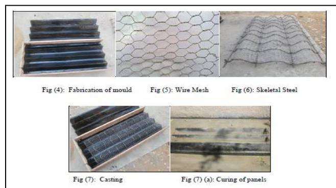
**Figure.1** Casting and curing of folded panels
