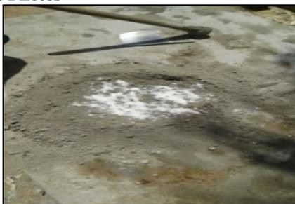
**Figure. 9** At The Stage Of Chemicals Addition (NaOH & Na<sub>2</sub>SiO<sub>3</sub>)
