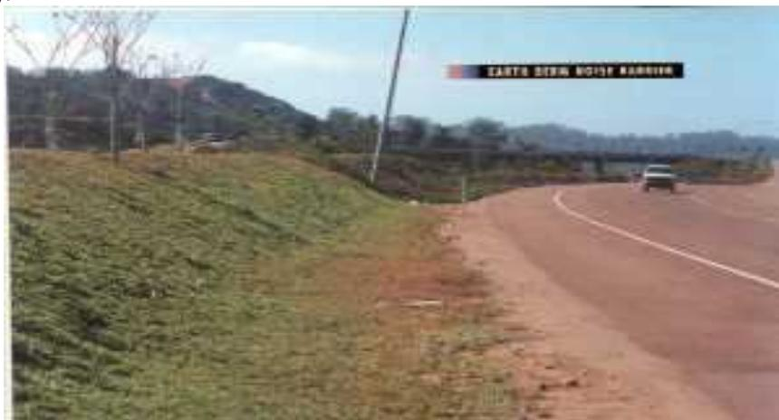
**Figure 4.4:** Earth noise barrier
