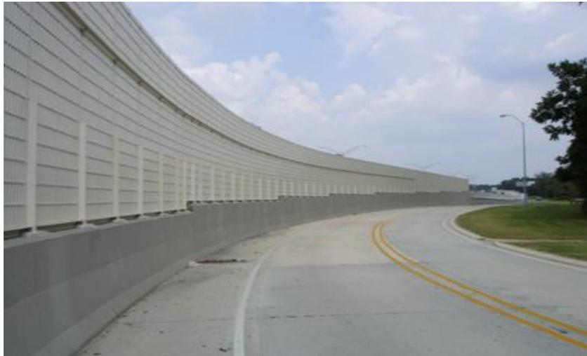
**Figure 4.6:** Concrete Noise Barrier with Wood grain Texture Noise Barrier Examples
