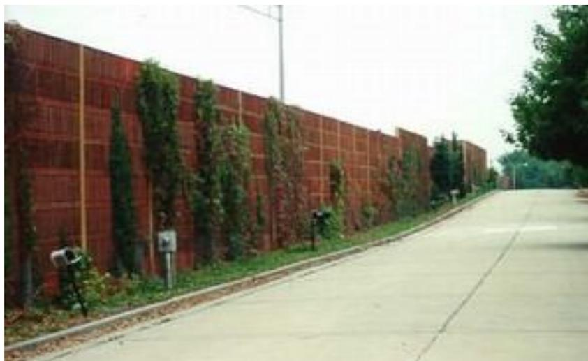
**Figure 4.5:** Wooden Noise Barrier
