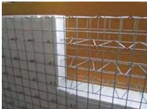
**Figure 3** Welded reinforcing mesh 3-D panel without expanded polystyrene
